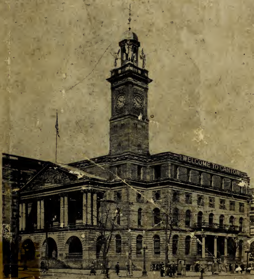
STARK COUNTY COURT HOUSE, CANTON
